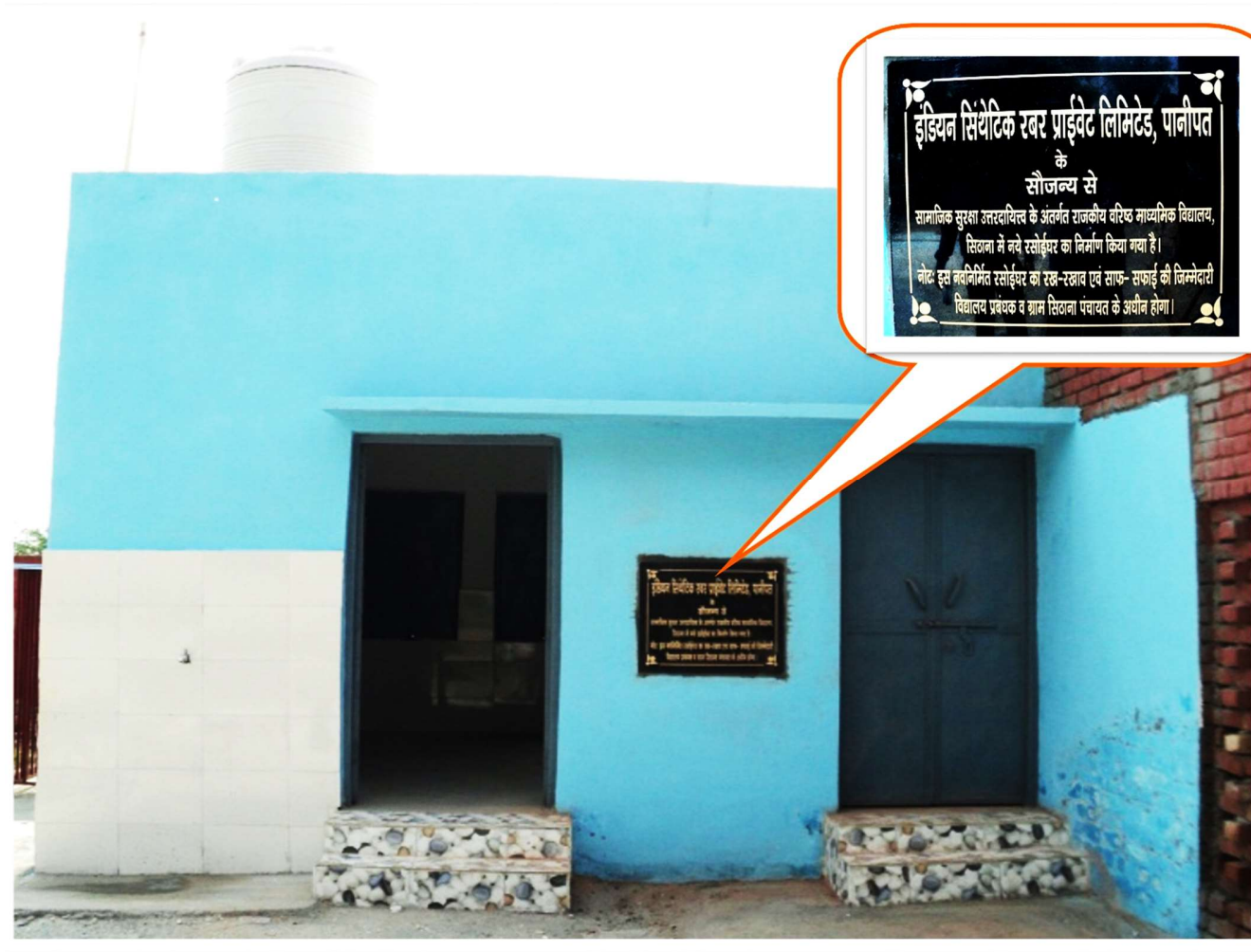
To facilitate Mid-day Meal Preparation for children's of School a New Kitchen Constructed at Govt. Sr. Sec School Sithana, Panipat (Haryana) Under Promotion of education Scheme of CSR by ISRPL Panipat in FY 2019-20
